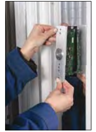
Remove sensor and install replacement unit.
